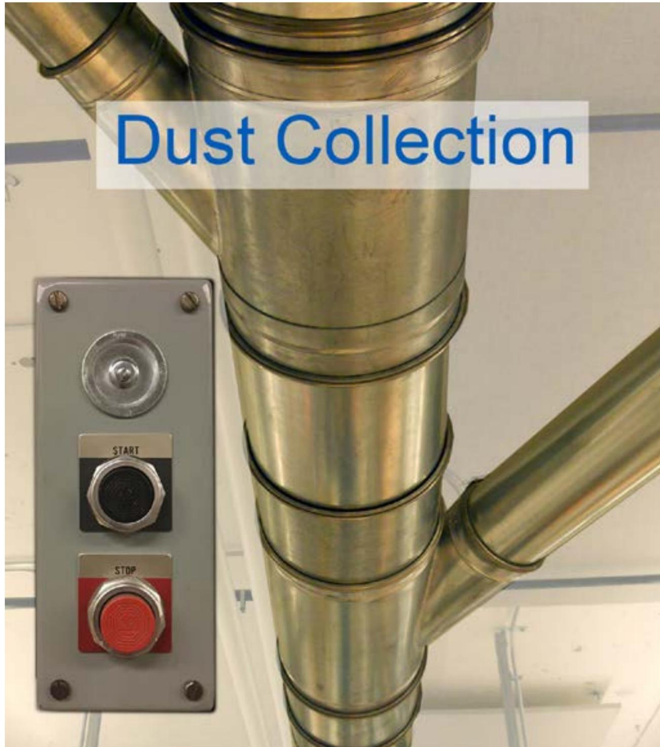
**Air Revolver-** This system captures harmful fumes and particulate and pulls them through filters. Fumes from cutting some plastic, for example, can be unhealthy.
